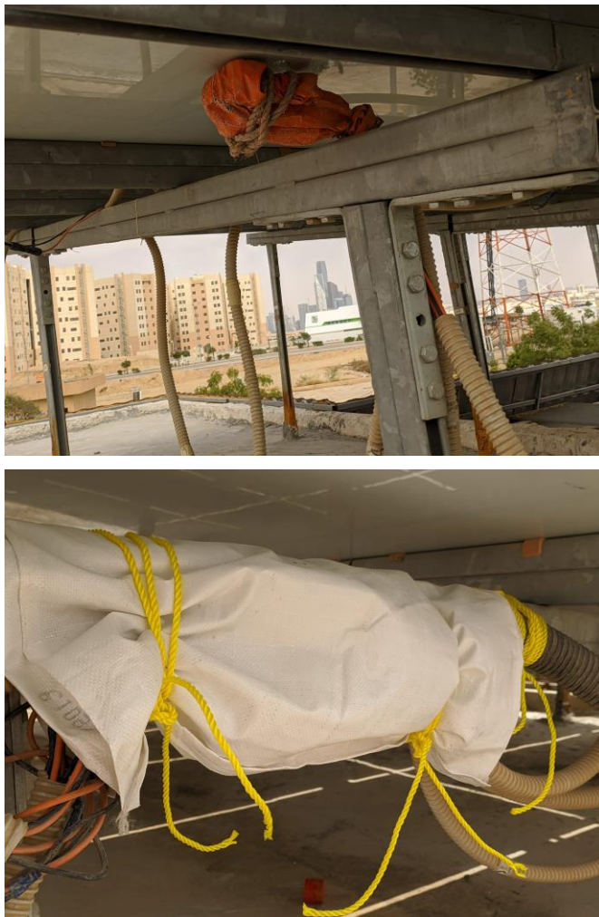
Figure 3.13 String cables after repair
