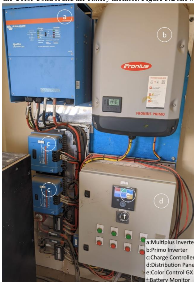
Figure 3.1 The north wall of the technical room
