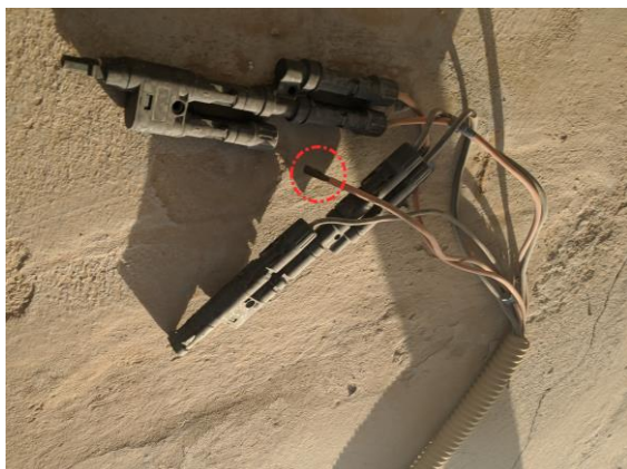
Figure 3.5 A disconnected string cable
