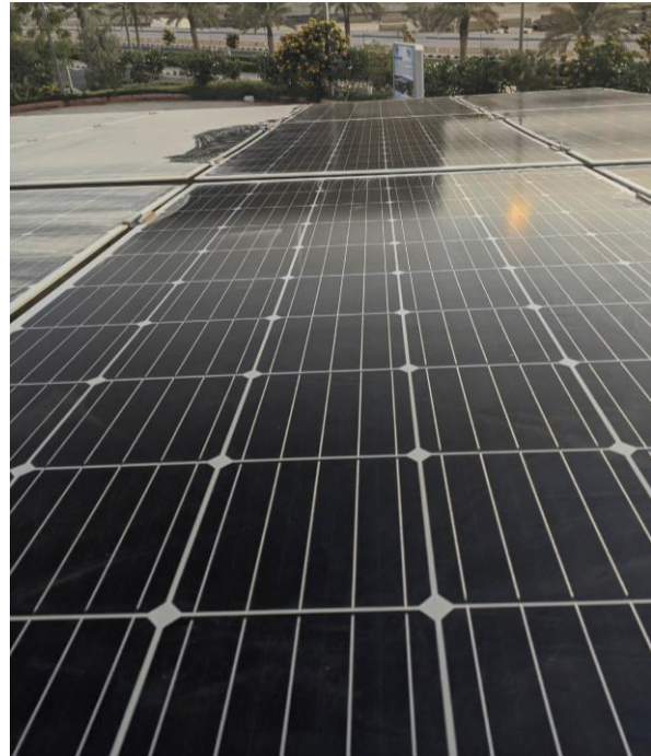
Figure 3.8 The solar modules during cleaning
