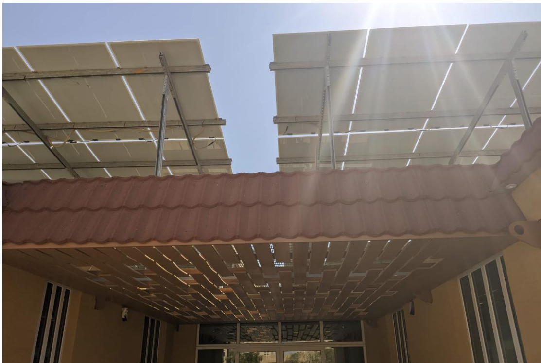
Figure 7.5 Picture showing the shading provided by the PV array
