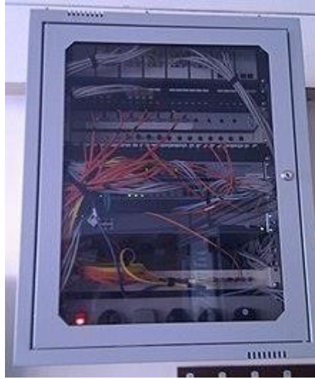
Figure 2.3: An Optical fiber junction box
